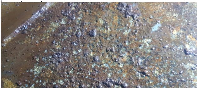
Corroded tank surface before Woltank Austria operation
