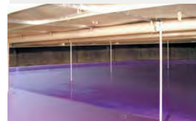
Figure 4. Double floor technology based on epoxy coating
