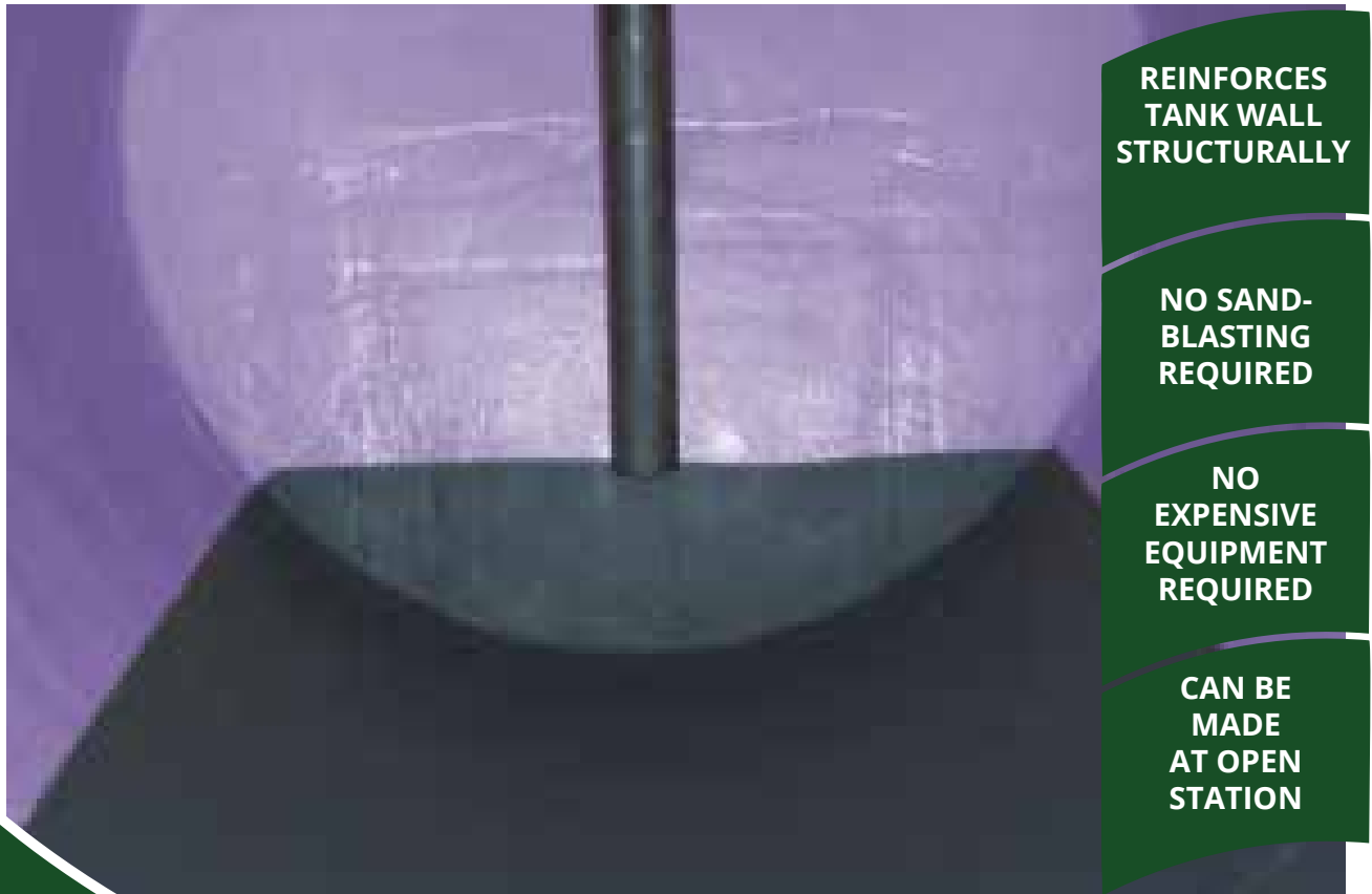
Applied EPOFLEX® tank lining in an underground storage tank i
