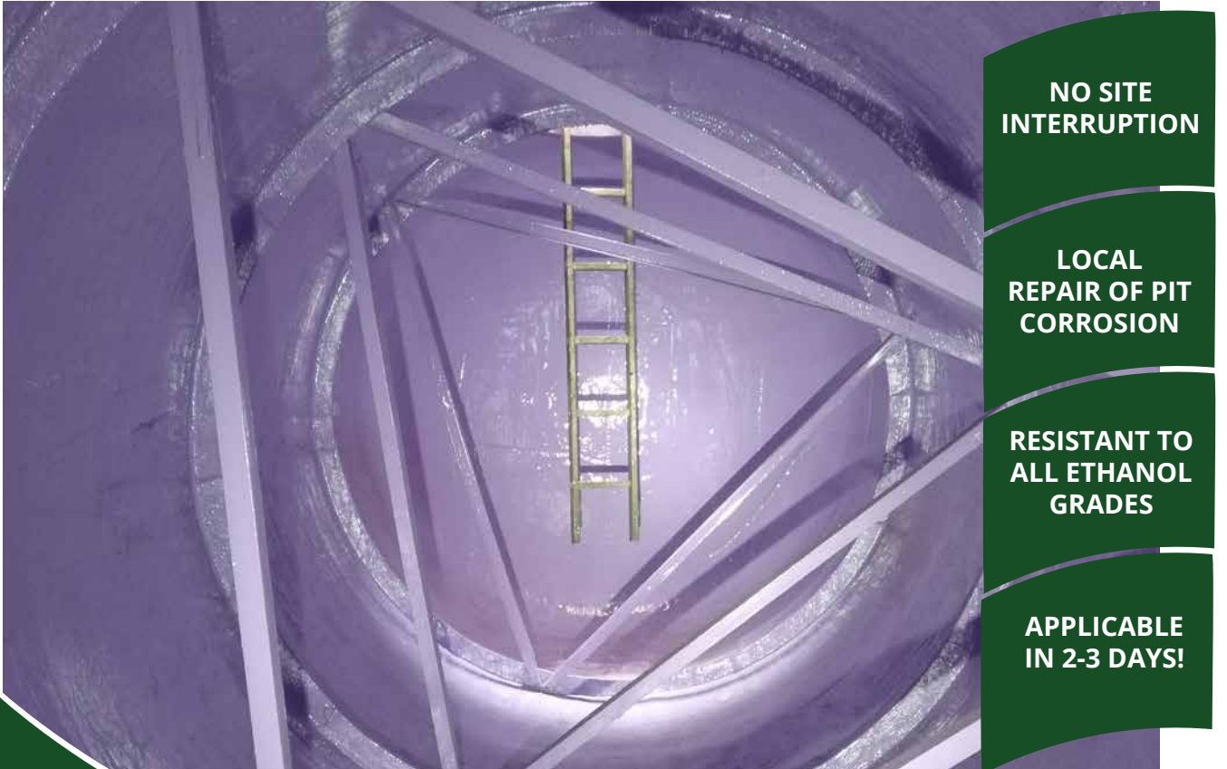
Reinforced tank completely protected with EPOFLEX® tank lining i
