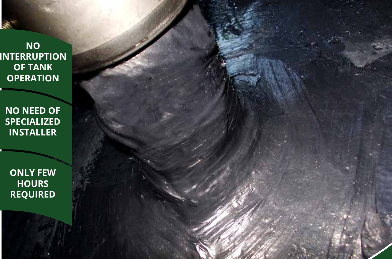
i EPOFLEX® DOM sealing applied and restored basic functionality
